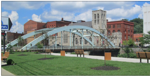
View of Center Street Bridge in Oil City.
