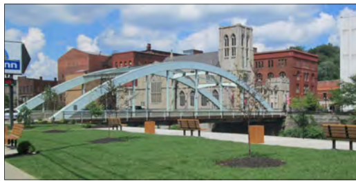
View of Center Street Bridge in Oil City.
