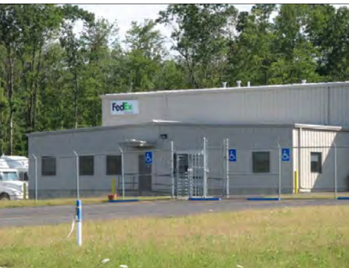
Fed Ex new construction in the SIP.
