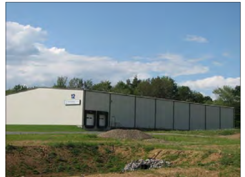
Latrobe Steel facility in the SIP.
