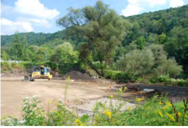
Figure 8. Oil Creek Memorial Landing under construction in September, 2015
