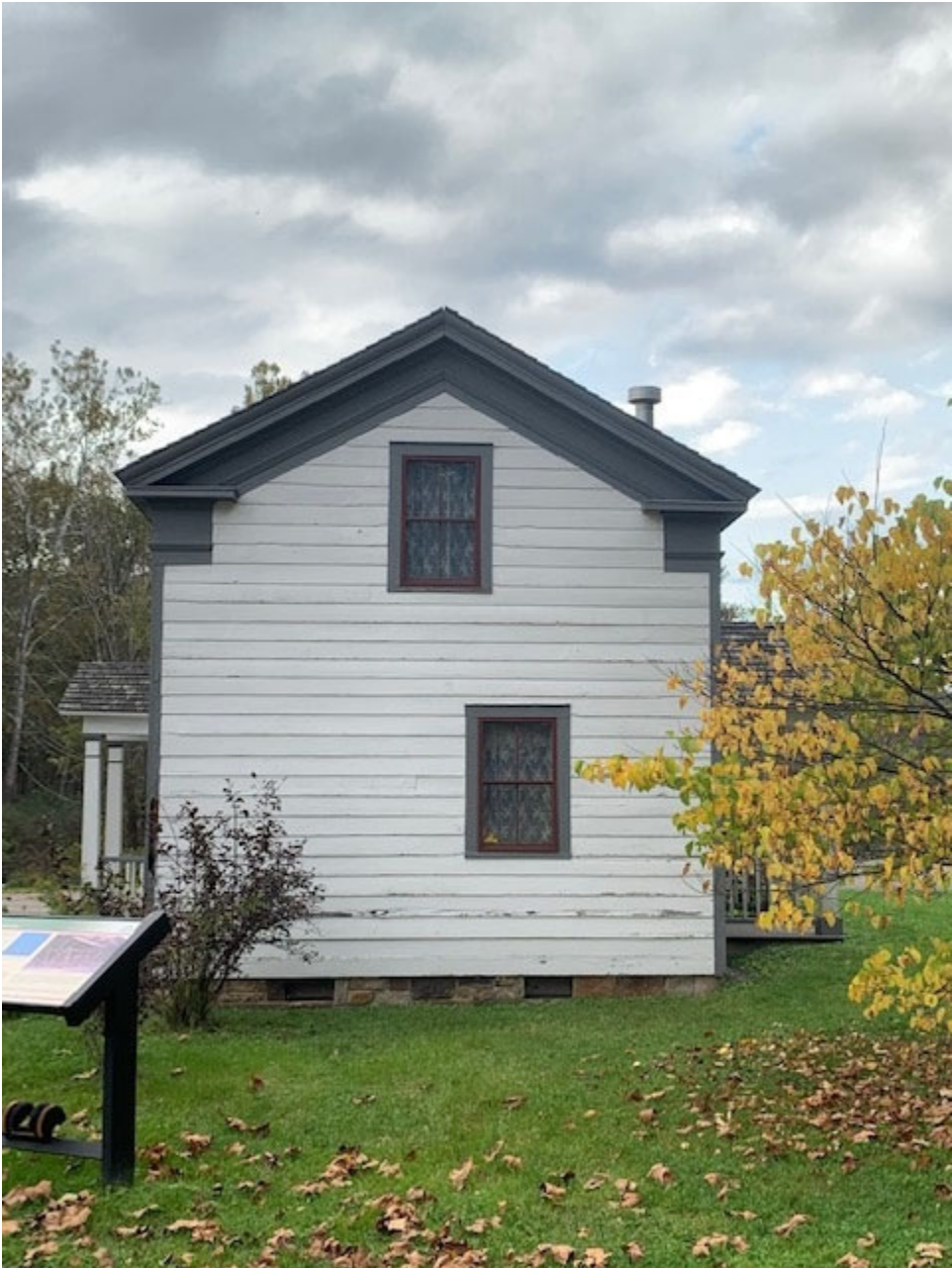
Right Elevation, Facing Parking Lot:
