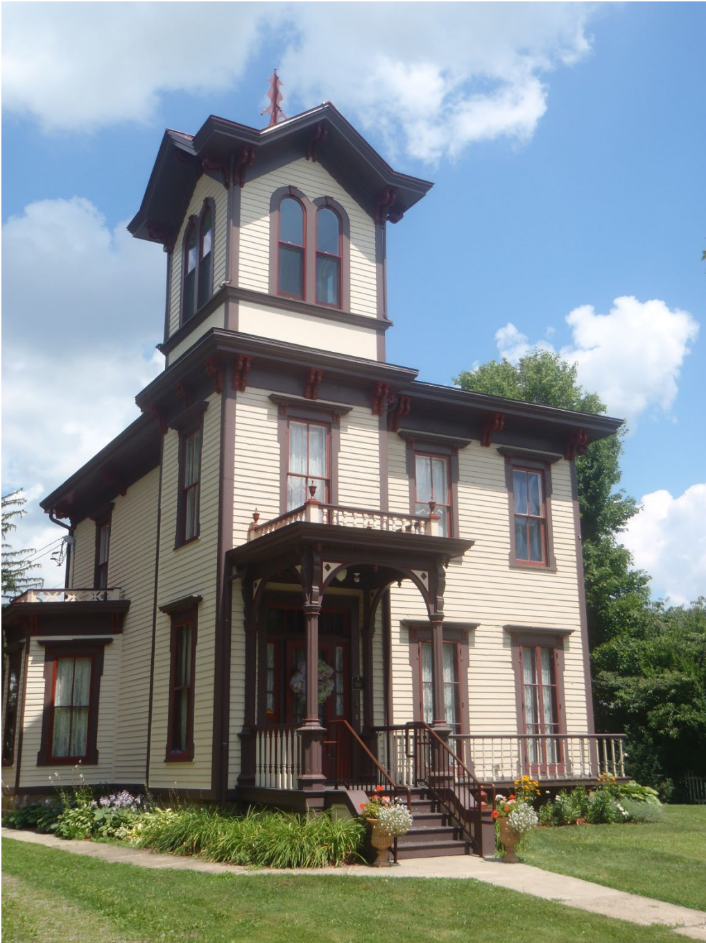
Tarbell House after completed Restoration Work, Front Elevation
