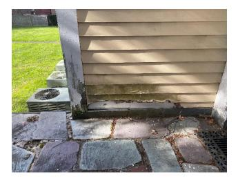
Replacement of damaged siding, stone base, and section of rotten corner board.
