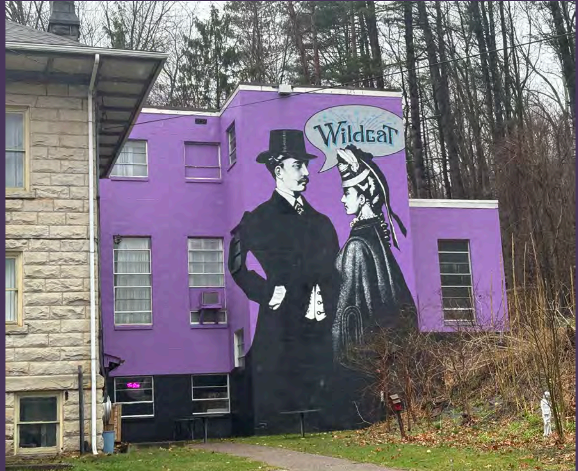
Rear Addition After
