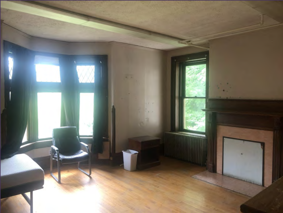
Terra Cotta Room Before
