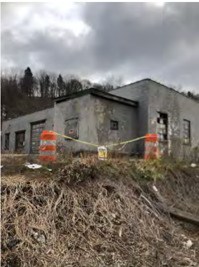
Photograph 13: Rear side of concrete block manufacturing building.
