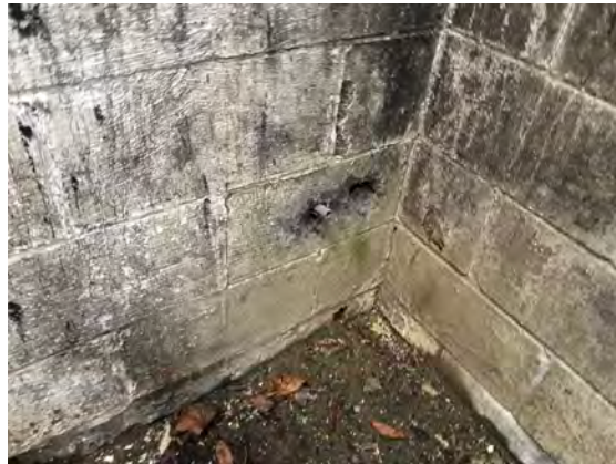
Photograph 8: Piping from UST outside concrete block manufacturing building.
