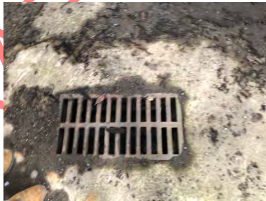
Photograph 10: Drain in concrete block manufacturing building.
