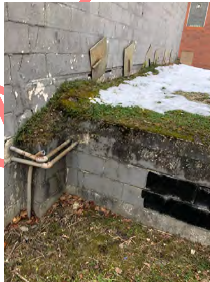
Photograph 4: Vent pipes of UST outside concrete block manufacturing building.
