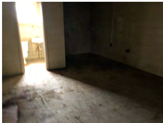
Photograph 6: Office space and bathroom.
