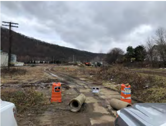
Photograph 1: Entrance from Duncomb Street looking south
