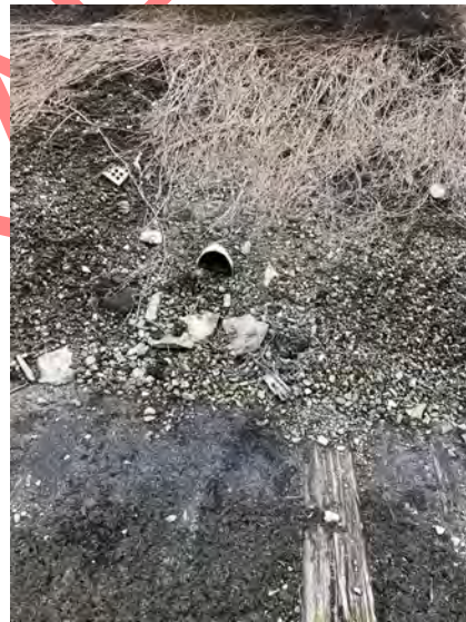
Photograph 14: Drain pipe on railroad.
