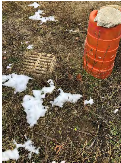
Photograph 74: Drain in center of subject site.
