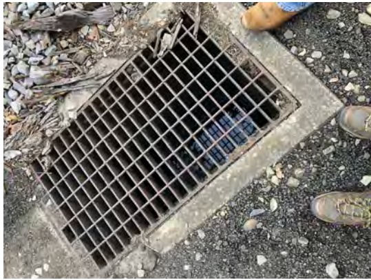
Photograph 15: Sewer grate for public water supply along railroad.
