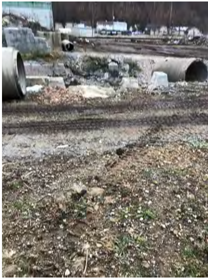
Photograph 39: Trench and old materials for concrete manufacturing.
