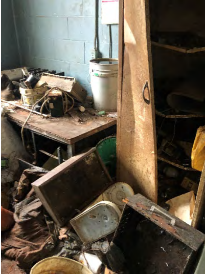
Photograph 81: Debris inside Dahlstrom office.
