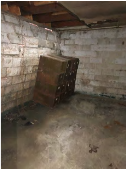
Photograph 27: Rear room in former dry-cleaning building.
