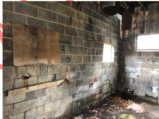
Photograph 36: Inside of boiler room building.
