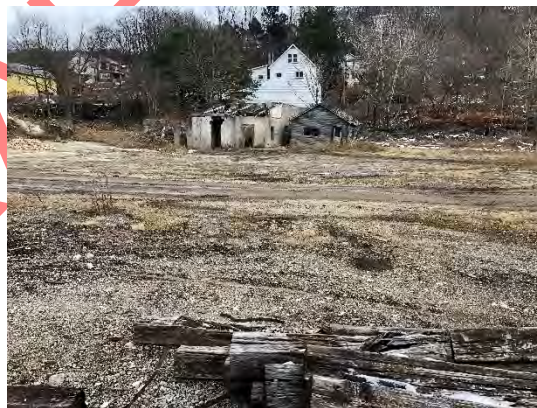
Photograph 80: Stained soils on Kraft property looking east towards office and boiler room building.
