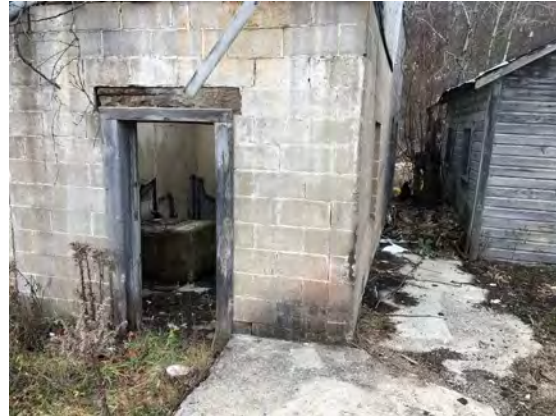
Photograph 34: Boiler room building (left), office (right)
