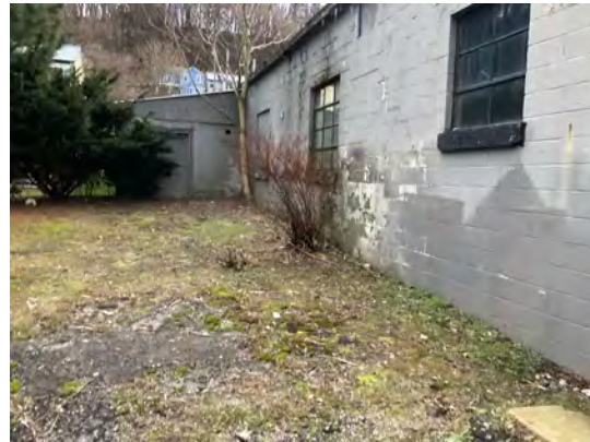
Photograph 28: Rear of former dry-cleaning building.
