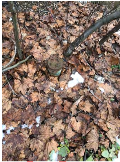
Photograph 38: Fill pipe for UST outside boiler room building.
