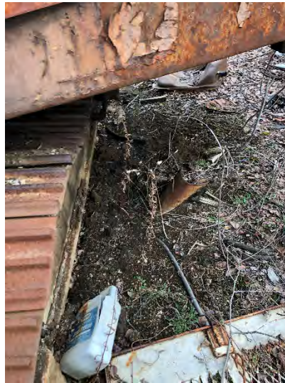
Photograph 102: Staining around scrap yard equipment.
