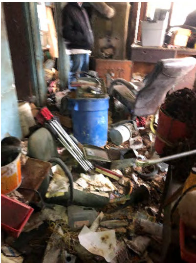
Photograph 83: Debris inside Dahlstrom office.
