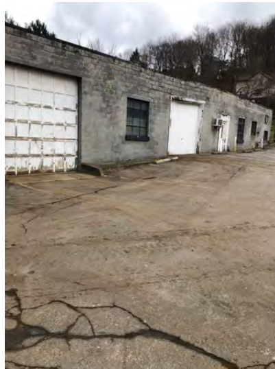
Photograph 16: Former dry-cleaning building.
