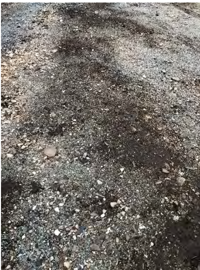
Photograph 75: Stained soils on Kraft and Dahlstrom property.
