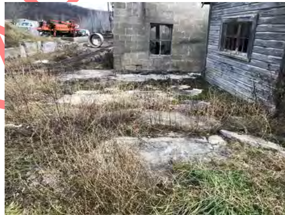
Photograph 30: Office and boiler room building.
