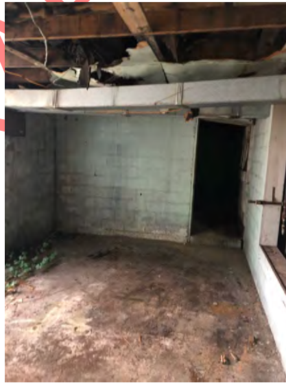
Photograph 26: Rear room in former dry-cleaning building.
