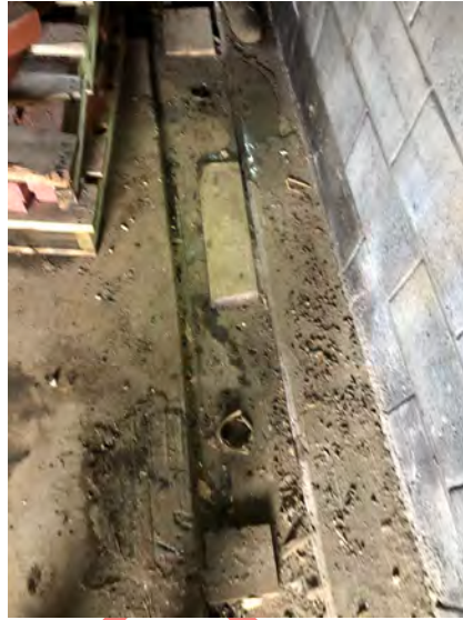
Photograph 20: Drainage features in former dry-cleaning building.
