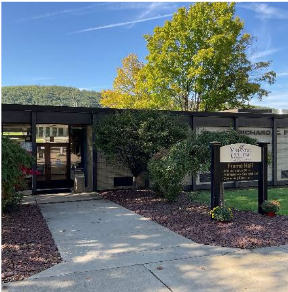
Frame Hall front entrance
