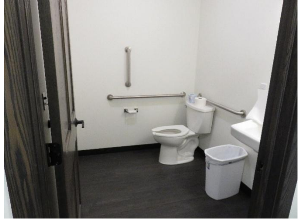
Finished First Floor ADA Restroom
