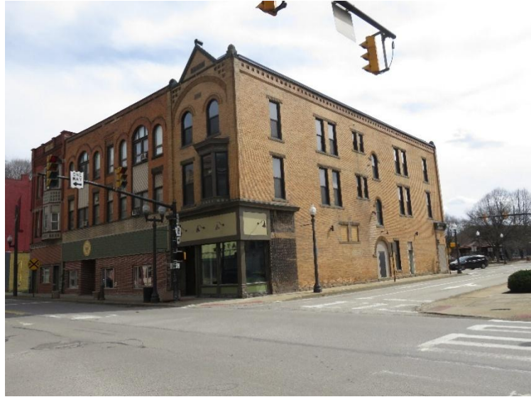
North Façade (left), West Façade (right). Intersection of Elm Street and Central Street.
