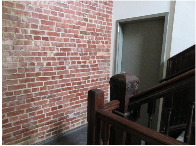
Stair Landing at Second Floor
